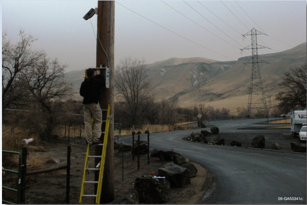
Each weather station measures and records wind speed peaks, wind speed averages, wind direction averages, temperature, as well as operating battery voltage.
